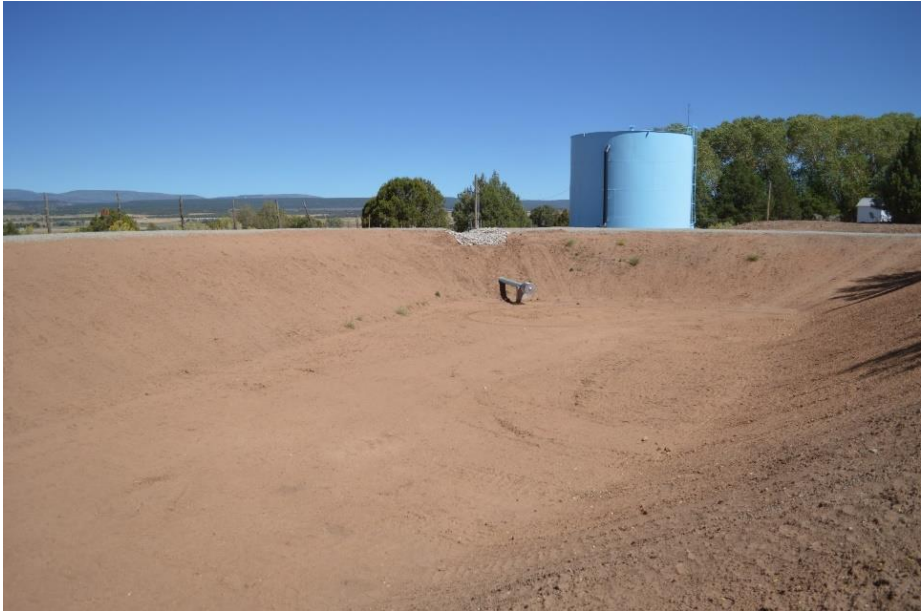
Figure 2-8 Raw Water Reservoir before filling
