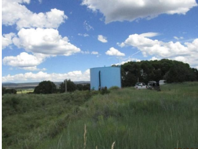
Figure 2-6 200,000 Gallon Blue Tank
